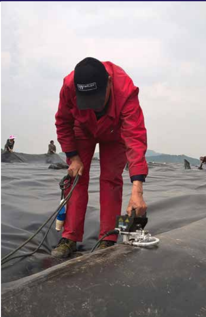
Hot wedge, 56 x 36 mm, copper with test channel 156.617
